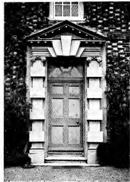
DOOR AT STANFORD DINGLEY
